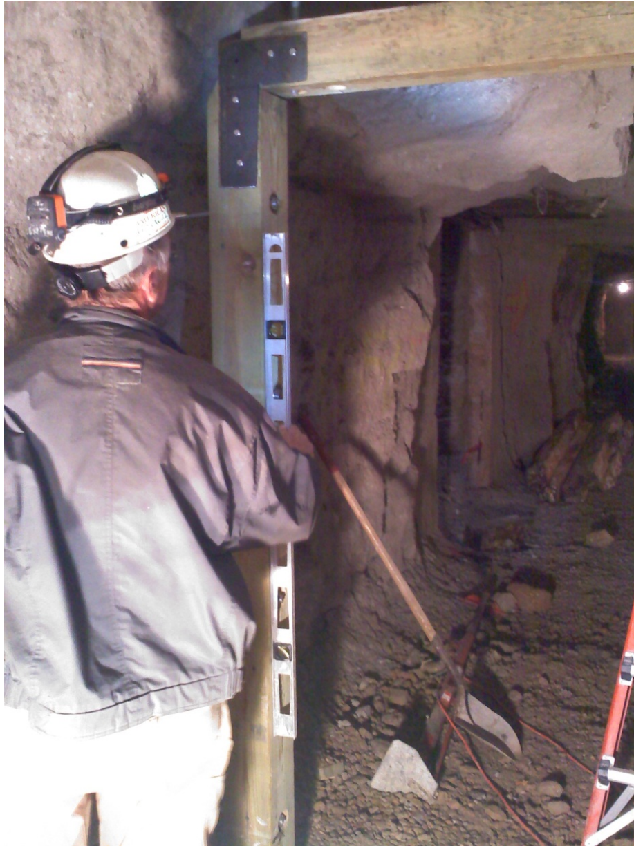
Figure 7.11. Steel plate attached to frame pieces
